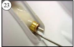
Scoop out any epoxy under the end of the Stern Tube.
