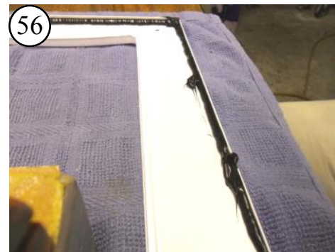
56 It doesn't have to be pretty. Fill evenly and wipe off any excess. Note how the sealant is pressed into the corner.
