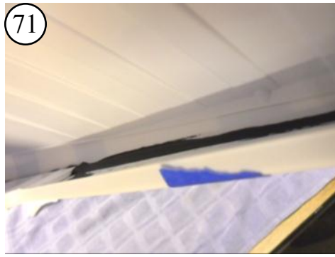
71 Smoothed sealant. Wider seal joint.
