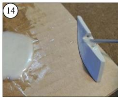
Put the filled epoxy on the bottom surfaces of the Skeg Reinforcement.
